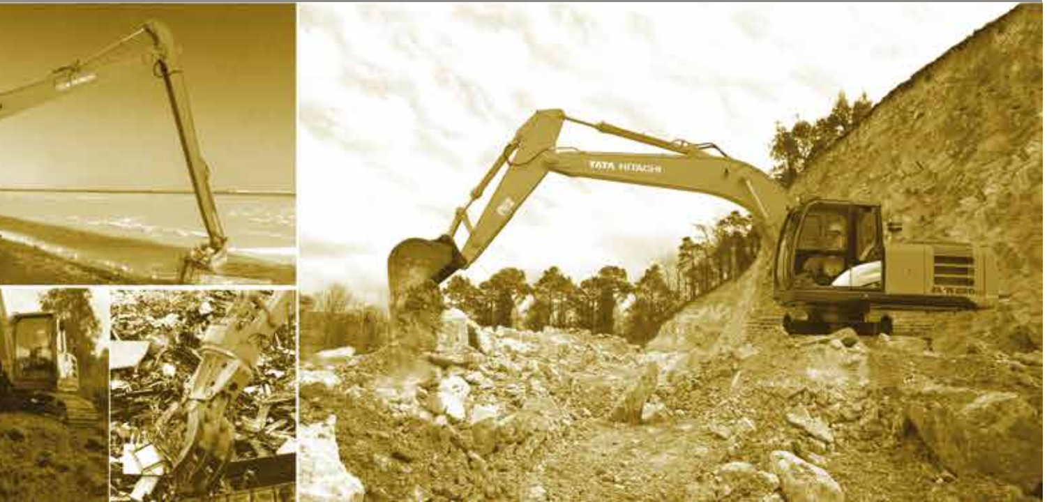
The photos above show machine images at work, which include machines other than ZAXIS 220LC-M
